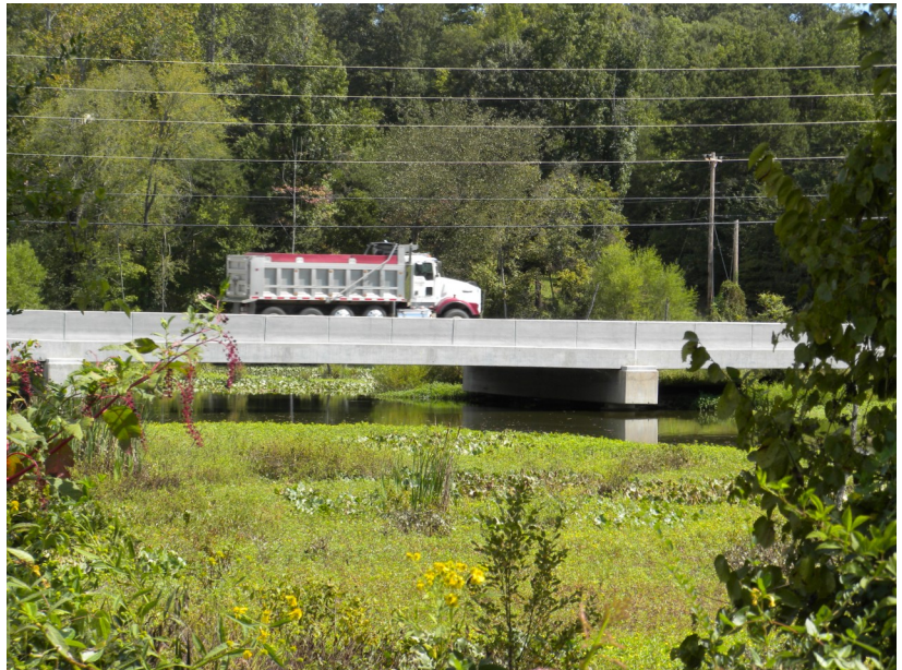
ARRA funds enabled NCDOT to build this new bridge on N.C. 73 over Long Creek in Albemarle (Stanly County). It replaces a 97 year old bridge that was the fourth oldest in the State still in use.
